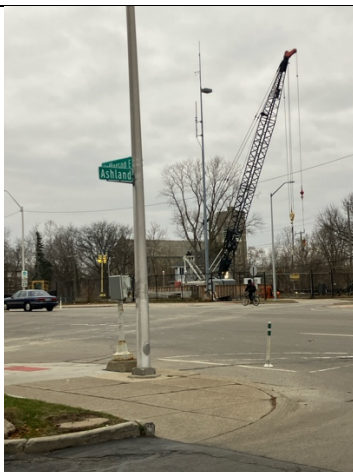
Cranes at Fox Creek Gates
