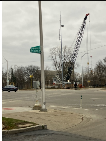
Cranes at Fox Creek Gates
