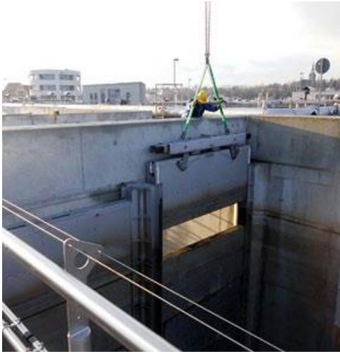
Figure 4. stoplog structure
